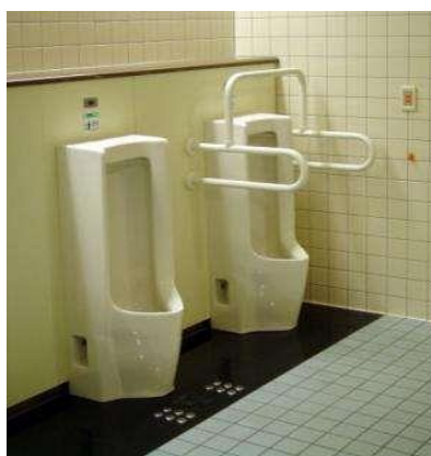
Photo 15-1. Floor Markings with Warning Pavers for Persons with Visual Impairments
