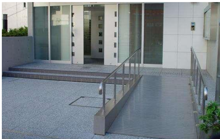
Photo 7.1 Combination of ramp and steps
