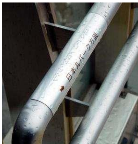
Photo 9-1. Handrail with Braille Information
