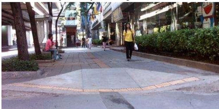
Photo 2-1. Step less entry with Designated Accessible Parking
